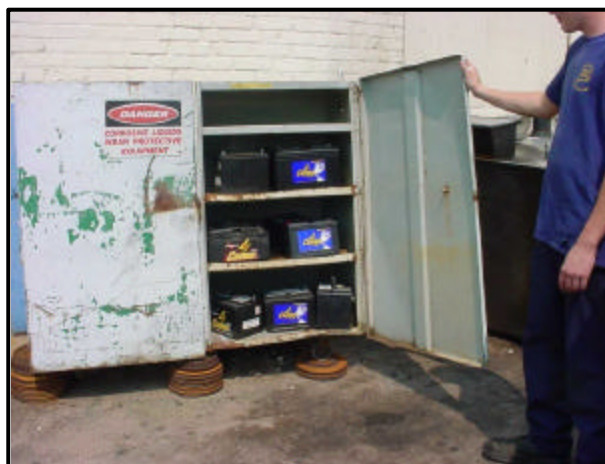
Batteries protected from the elements
