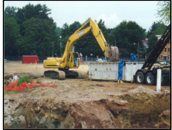
Removal of soil contaminated by a leaking underground storage tank
